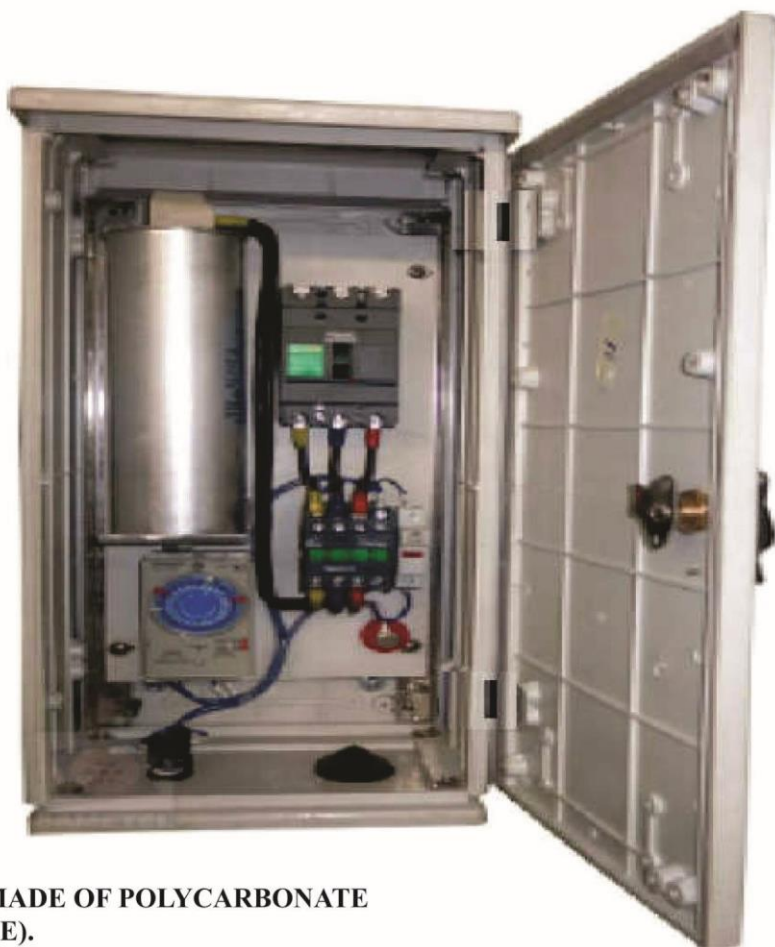
A2 – Pilar Electrical Cabinet, Electrical Distribution Cabinet and Capacitance Compensation Cabinet.
